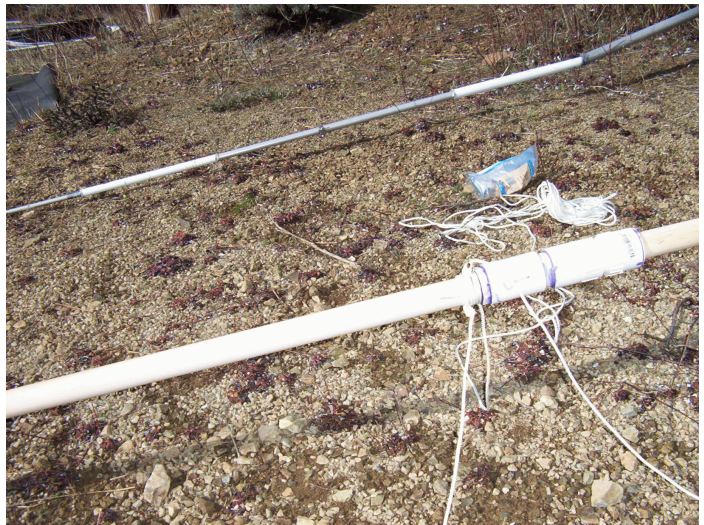
The PVC pipes fastened together over the antenna coupler, with cord guys attached.
